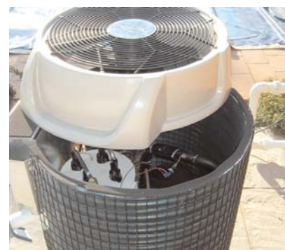
Remove top fan housing to gain access to high/low limit switches
